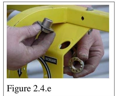
5. Install pressure gauges onto pressure gauge plate.
